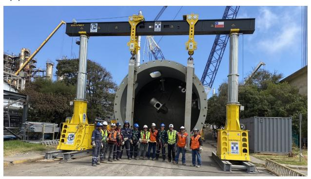
In late November, Engineered Rigging's heavy lifting experts mobilized the SBL500 from the Santiago yard. The team assembled the gantry, which features an octagonal boom for added strength and increased capacity and lifting height. Using the gantry's Intelli-Lift wireless control system, the operator remotely lifted the scrubber from DSV's specialized transport system and lowered it onto static storage stands. ER's team then disassembled the gantry and returned with it to Santiago.
