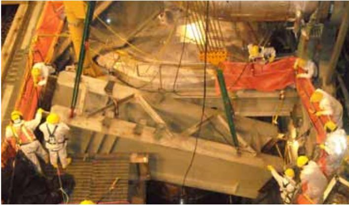
When an Engineered Rigging team set out to perform a motor changeout for an industrial plant in Arkansas, it could have used conventional scaffolding for the job. But one team member had a better idea: Deploy portable, lightweight construction platforms called Angel Wings to support workers performing inspection, repair and “hot work” tasks such as welding and cutting.
