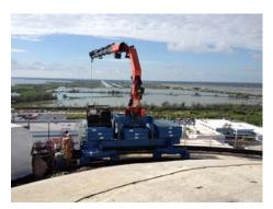
First, they needed to identify a staging area for the equipment and materials. Because there wasn't space on the ground, the rooftop of the adjacent building was the only option. Quite literally rising to the occasion, the company's engineers designed a highly maneuverable transport system by fabricating a customized cart to ride on the existing crane rails that ran circumferentially around the building's roof. Once the cart was in place, Engineered Rigging mounted a knuckle boom crane to
