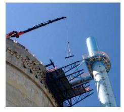
A testament to Engineered Rigging's commitment to safety and engineering prowess, the platform supported 10,000 lbs. of live load, plus 20,000 lbs. of self-weight, all without any support at the end. It was also strong enough to resist more than 30,000 lbs. in the horizontal direction.
